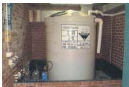
Figure 7 Bulk sodium hypochlorite container in bund
