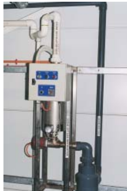
Figure 12 Ozone off-gas destructor
