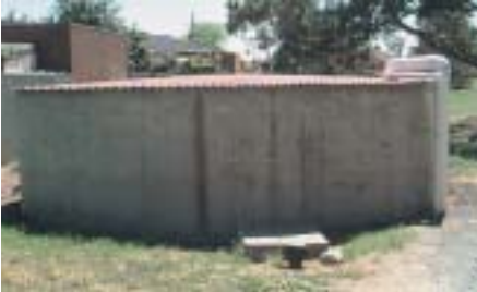
Figure 4 Backwash tank
