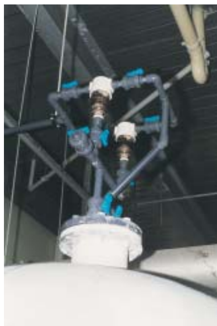
Figure 33 Filter off-gas bleed and collectors
