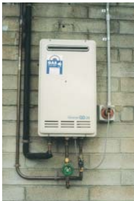
Figure 5 Instantaneous hot water system
