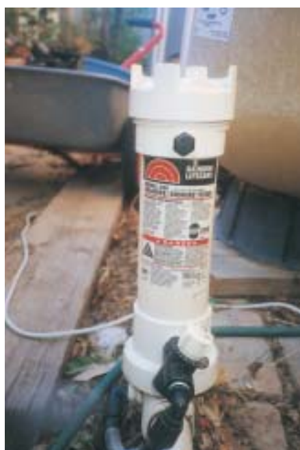
Figure 17 Erosion canister (erosion feeder)
