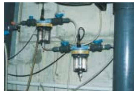
Figure 9 Pool water treatment with ozone and hypochlorite
