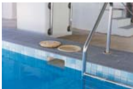
Figure 27 Skimmer box and lint trap
