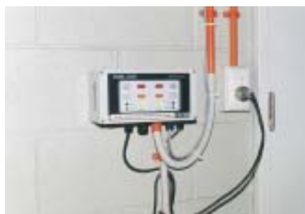
Figure 11 Ozone leak detector
