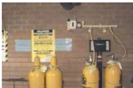
Figure 6 Chlorine gas, weight scales and regulator
