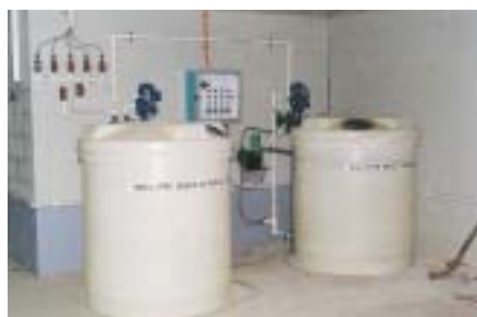
Figure 35 Dosing tanks with mixers for adding coagulant
