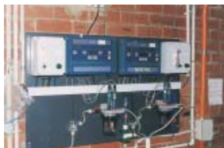
Figure 18 Pool control panel and chemical measuring station
