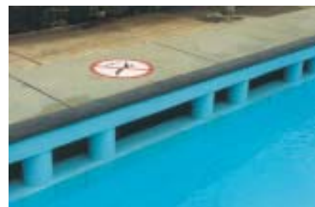
Figure 26 Overflow channel on an older outdoor pool
