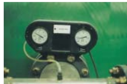
Figure 36 Pressure differential gauges
