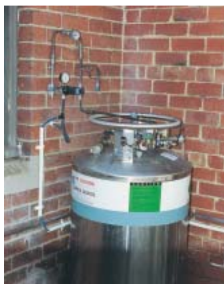
Figure 13 Carbon dioxide tank
